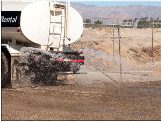
Easily Applied with Water Trucks!
