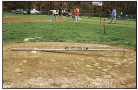
This simple tool can be made in a few minutes, and can help to set the correct slope toward home plate from the pitcher's plate.
