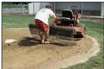
One of the secrets to correct dragging is to lift the drag before you leave the skinned area. Never drag skinned area soil into the grass, where it can affect drainage.
